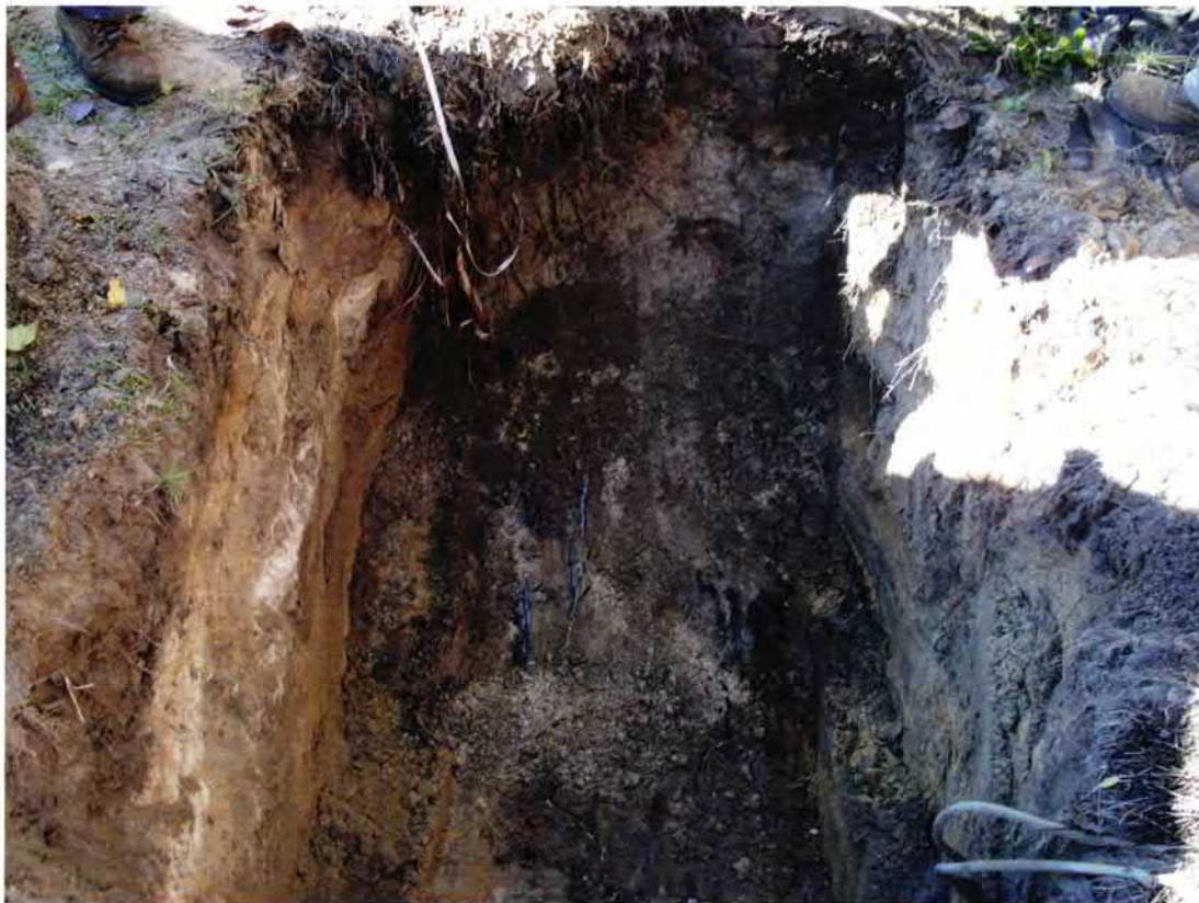
Picture 2: UST 892Cobia excavation.
